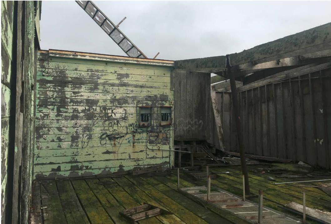
Due to the advanced deterioration, the pier was planned for removal. Removal of the pier and disposal upland would reduce the amount of chemically treated wood debris that is entering the ocean, thus alleviating environmental concerns.
