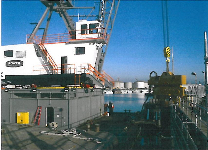
Figure 3 Barge Mounted Crane and Vibratory Hammer
