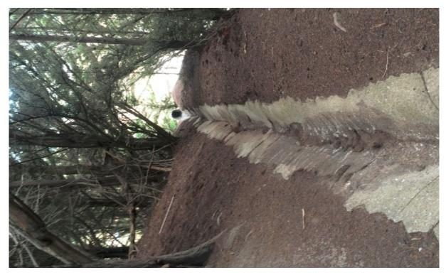
The upper concrete swale located on top of the adjacent bluff is in poor condition and is also to be addressed. The concrete swale channels rainwater from the bluff top to the mouth of a down pipe which terminates at an outfall culvert under the trail. The concrete swale has suffered damage in several locations, is to be repaired and the water re-directed to a nearby natural marsh wetlands.
