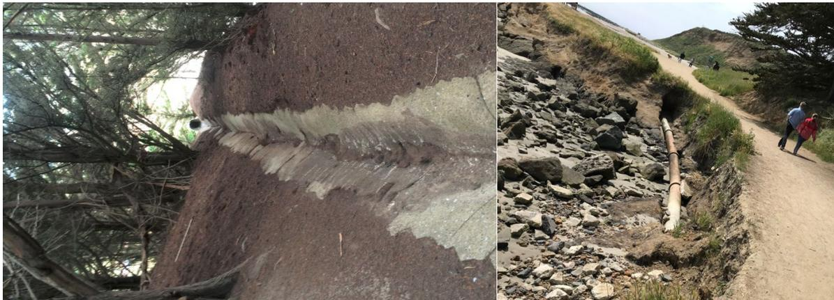
The upper concrete swale located on top of the adjacent bluff was also addressed. The concrete swale channels rainwater from the bluff top to the mouth of a down pipe which was replaced and covered. The upper swale now directs rainwater to a nearby natural marsh wetlands.
