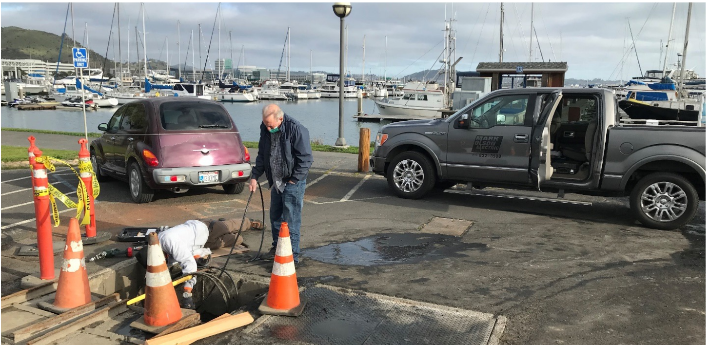
Figure 21. Oyster Point Marina – Electrical Pull Box Being Maintained to Dock 13
