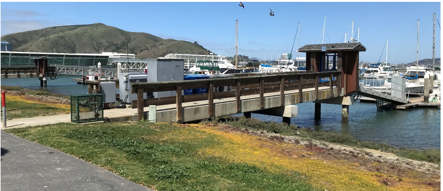
Figure 20. Oyster Point Marina – Landside Gangway Platform to Dock 12
