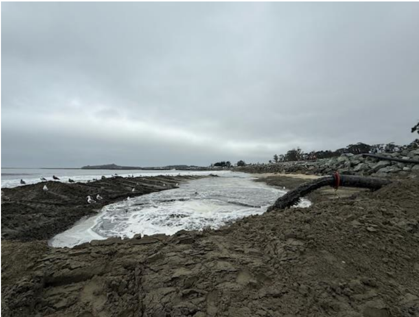
Northern containment cell on September 12, 2025
