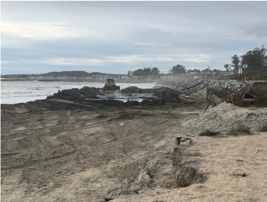
Sand placed on beach as of September 30, 2025
