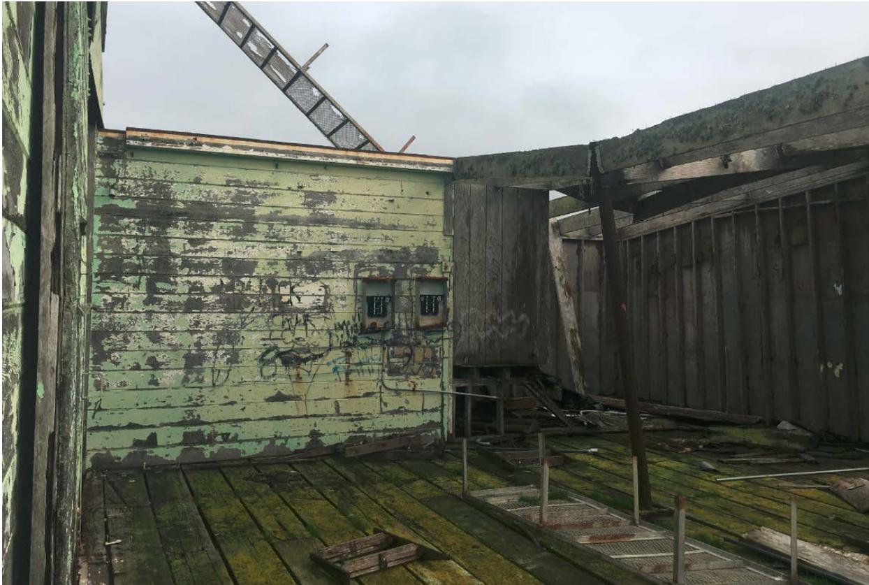
Due to the advanced deterioration, the pier was planned for removal. Removal of the pier and disposal upland will reduce the amount of chemically treated wood debris that is entering the ocean, thus alleviating environmental concerns.
