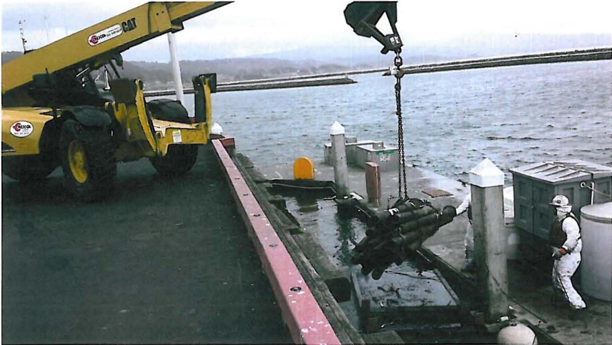
*Blue Pipe is the new sewer line using C900 pipe material with connection couplings at joints*
