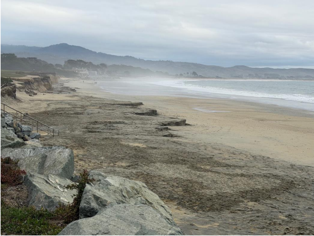
Completion of sand placement, October 31, 2025
