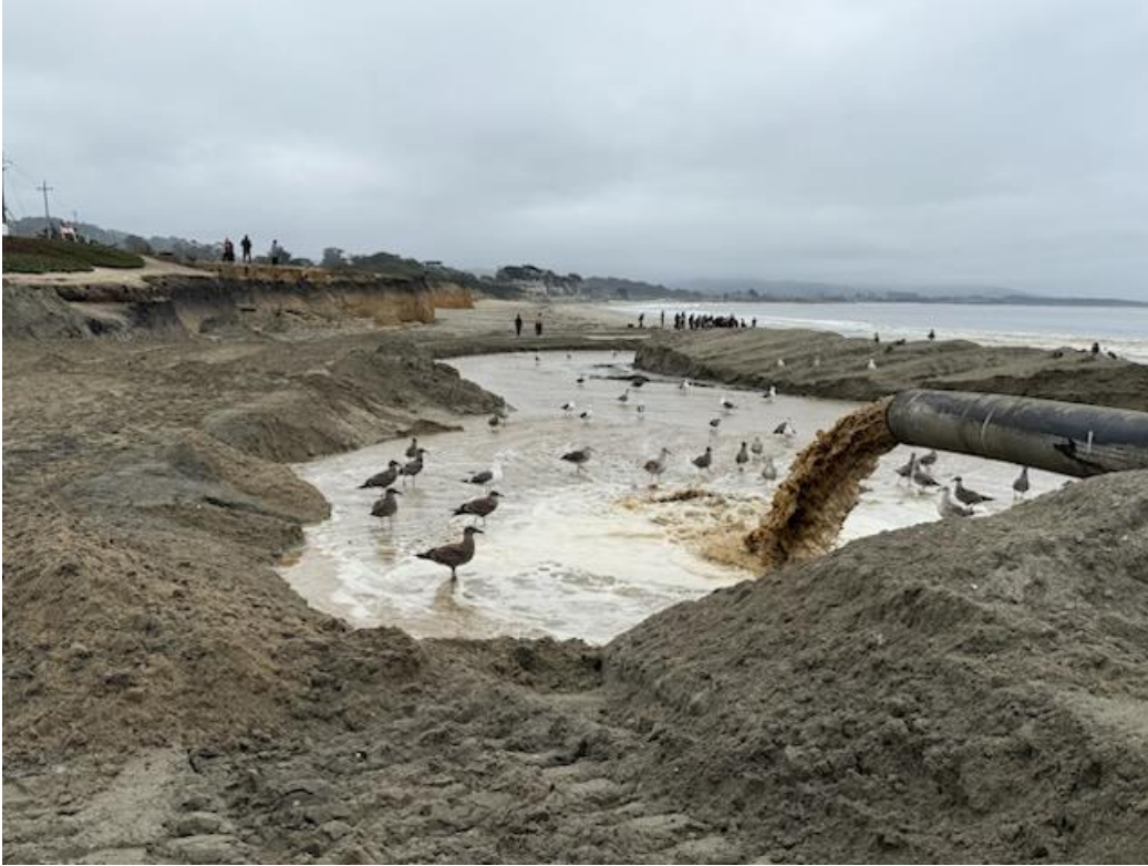
Southern containment cell on September 12, 2025
