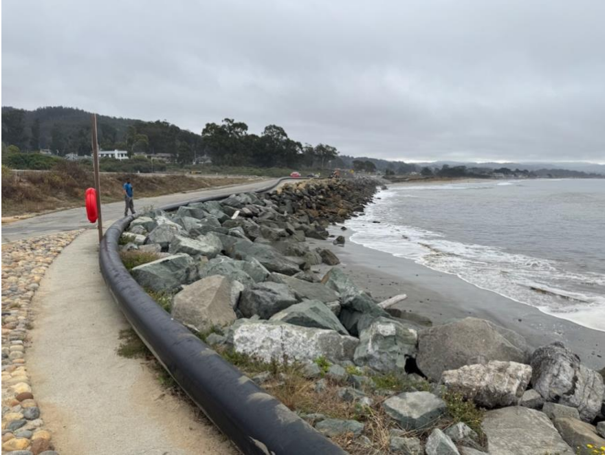
Pipeline alignment at Surfers Beach
