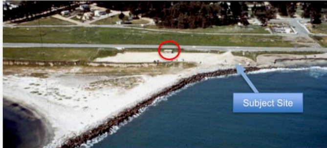
Figure 4. Subject Site, 1972 (California Coastal Records Project, Image 7217069)
