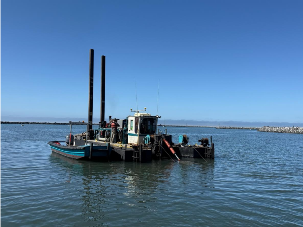
Dredging operations began on August 29, 2025
