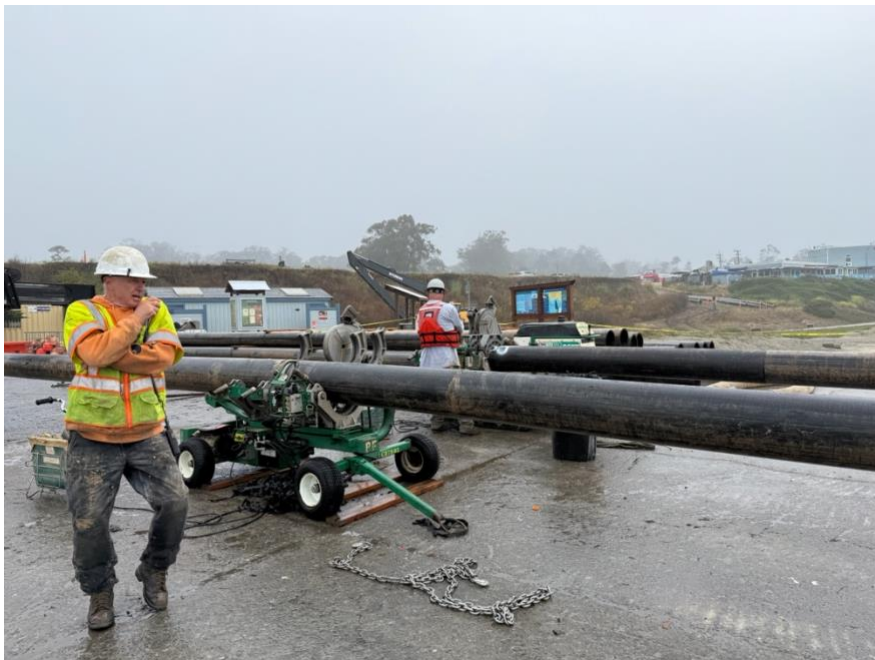
Dredge pipeline deployment at boat launch ramps
