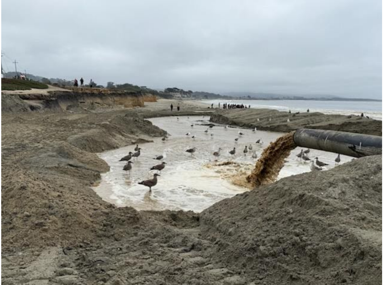
Southern containment cell on September 12, 2025
