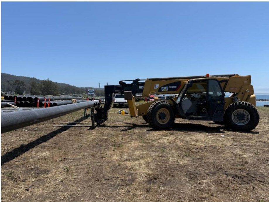
Telehandler for transporting pipe
