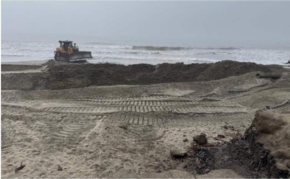
Pipeline alignment at Surfers Beach
