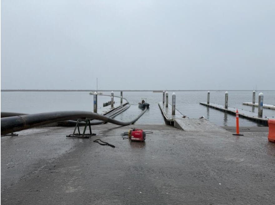
Dredge pipeline deployment at boat launch ramps
