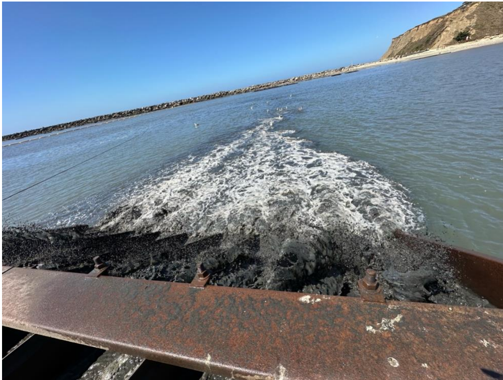
Placement of dredged sediment at eelgrass mitigation site, from placement barge
