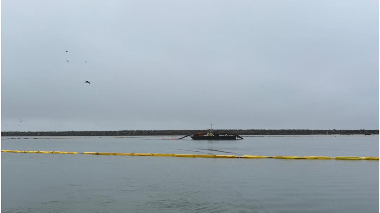
Placement barge depositing sediment within turbidity curtain at eelgrass mitigation area
