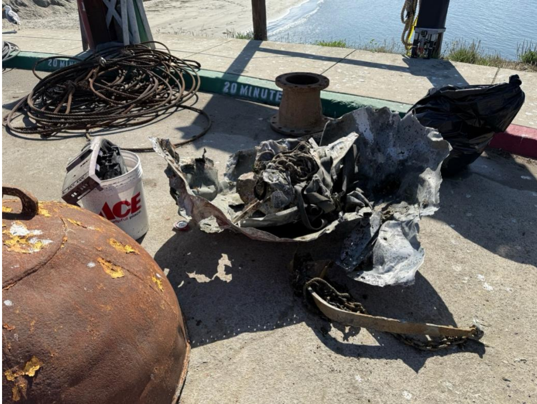
Debris encountered at Launch ramps while dredging
