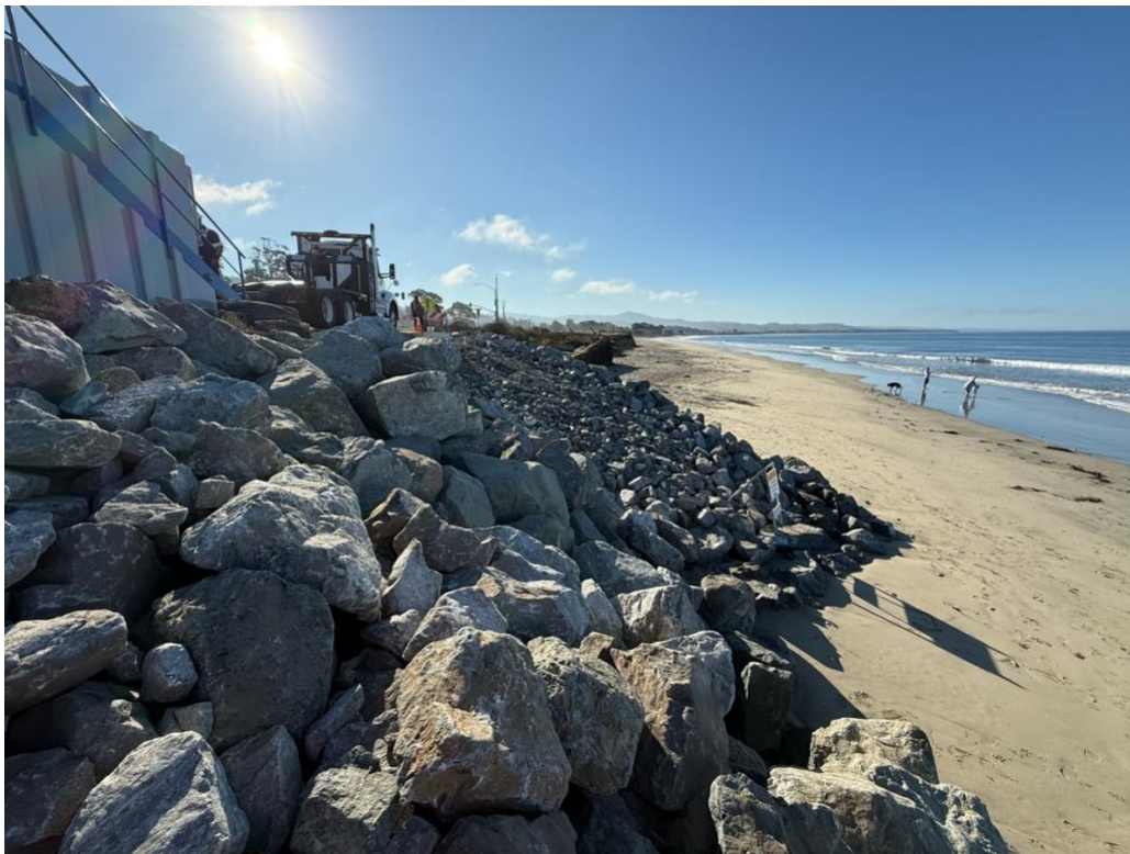
Temporary Heavy Equipment Access Ramp constructed at Surfers Beach
