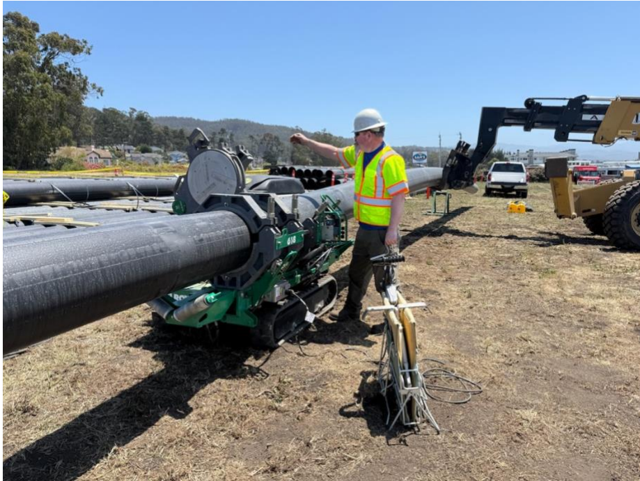
Dredge Pipeline Assembly
