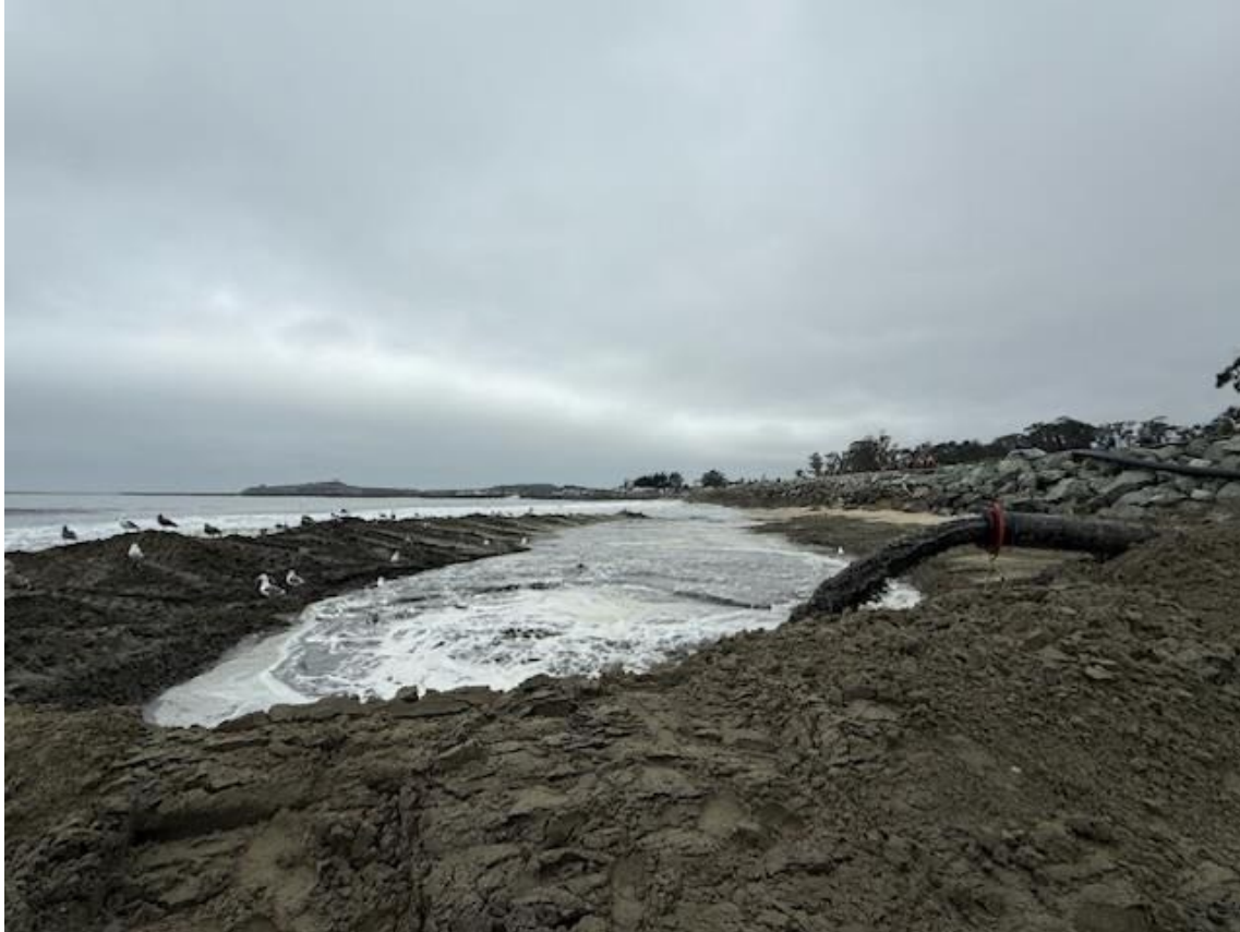
Northern containment cell on September 12, 2025
